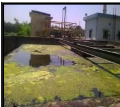
Figure 1: Algal source from Domestic Sewage Treatment Tank
