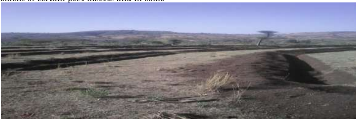
Figure 4: Soil bund constructed in the study area
