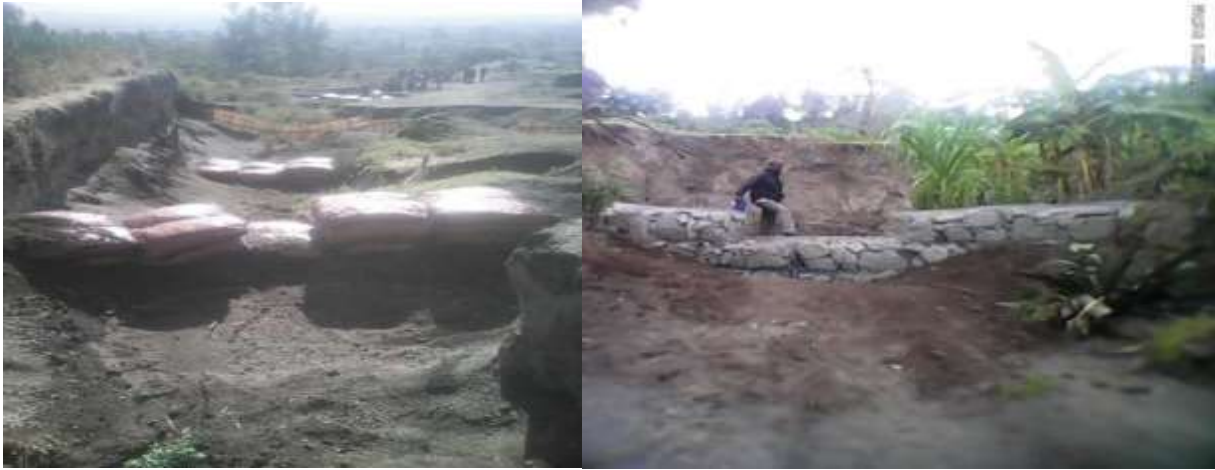
Figure 5: Check dam constructed on degraded communal land
